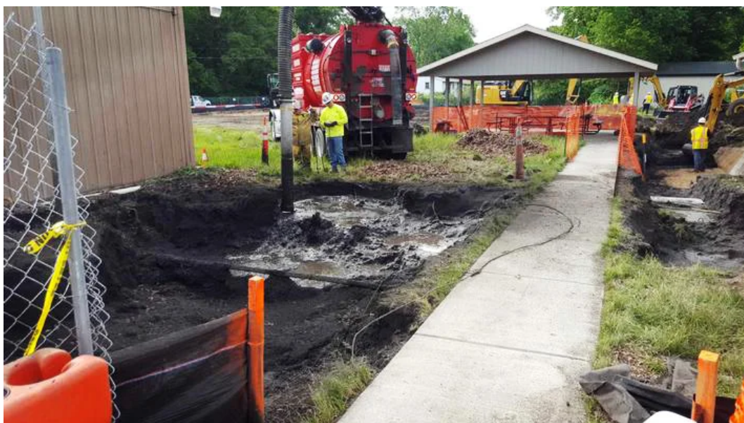
Vac truck excavation work near the town pavillion in Town of Pines, Indiana. (U.S. EPA)
